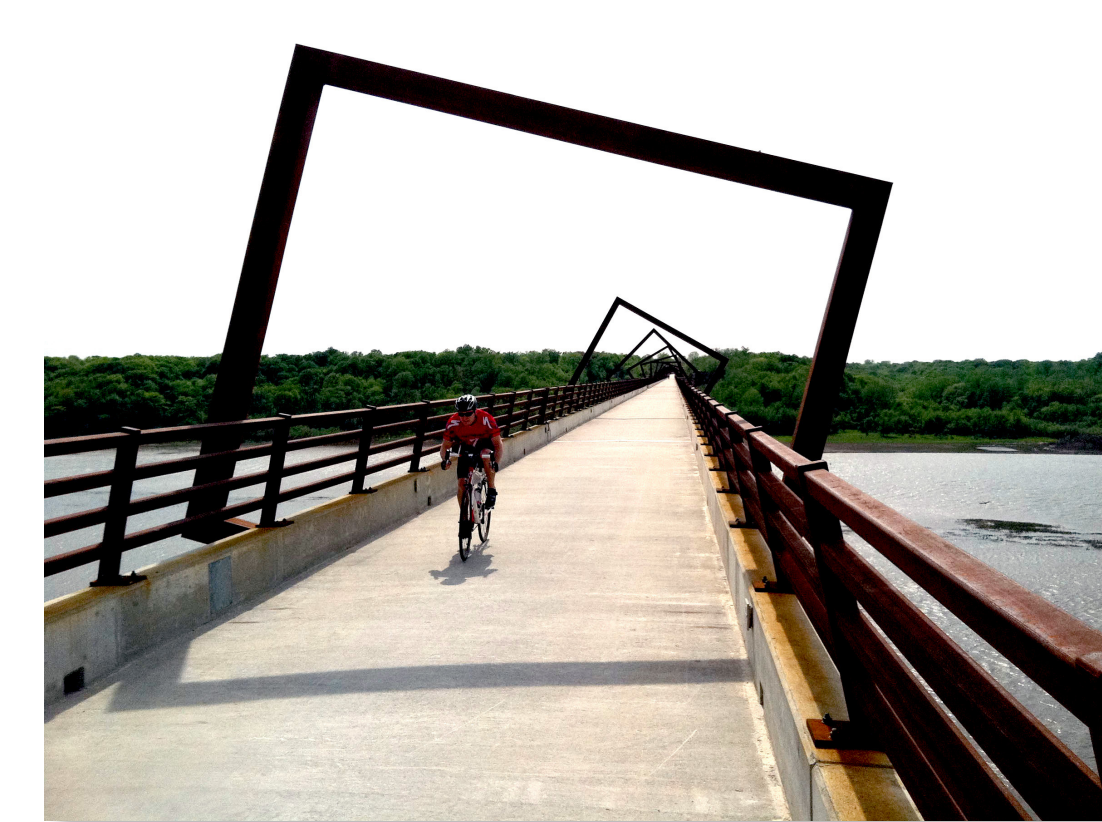
High Trestle Bridge. Source: Nate Schlorholtz
